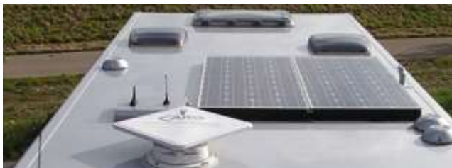
Installation Solarpanel 240W
